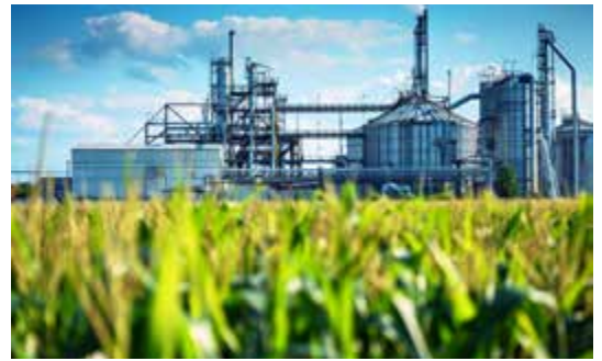
Biodiesel production plant
